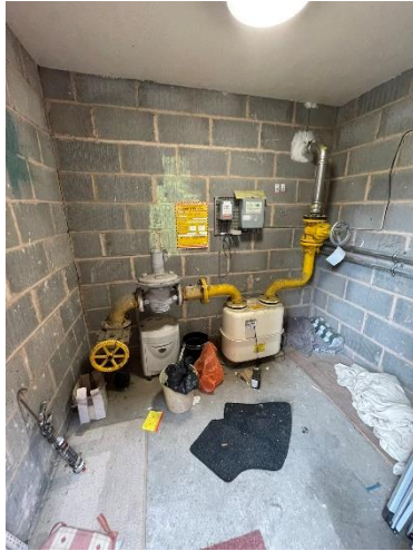
Gas Meter Room – Uninsulated Heating Pipework on Right Hand Side
