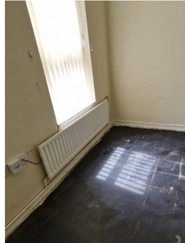
Example of Single Piped Radiator
