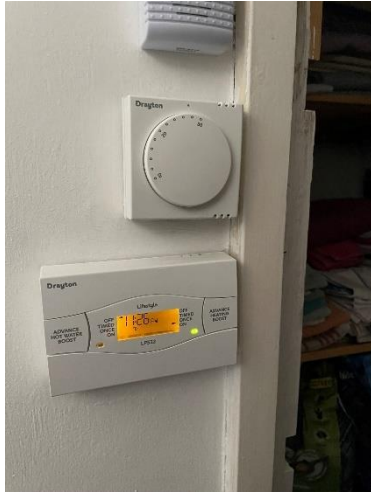
Thermostatic Controller (Set to 30°C)
